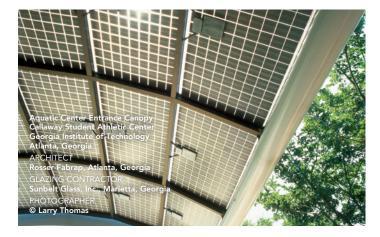
The polycrystalline PV panel consists of a piece of low-iron, tempered float glass. The solar cells are set between two layers of ethyl vinyl acetate (EVA) and laminated. The back of the ply or the interior side of the panel can be laminated with a protective layer of film. Overall panel thickness is 1/4".
